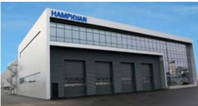
The Hampidjan Group headquarters are located at the waterfront of the main harbor of Reykjavik Iceland in a new 6.500 m2 building.
